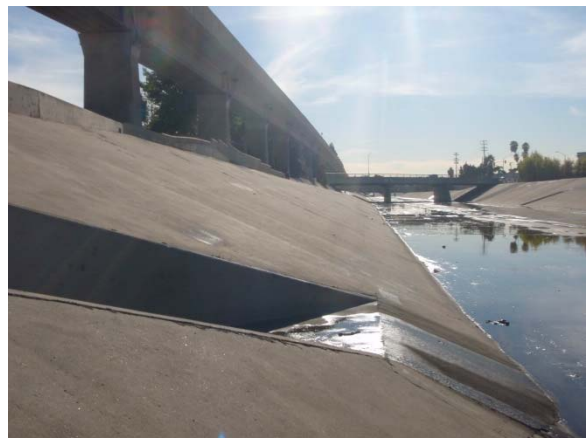
4. Looking south toward outfall
