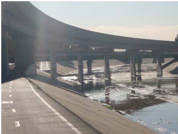
1. View of outfall north of railroad bridge
