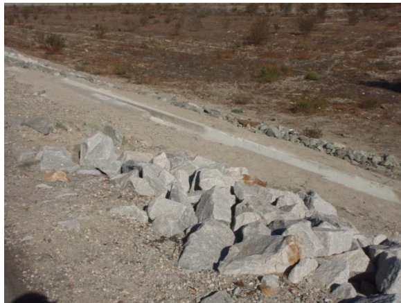
1. View looking down at outfall
