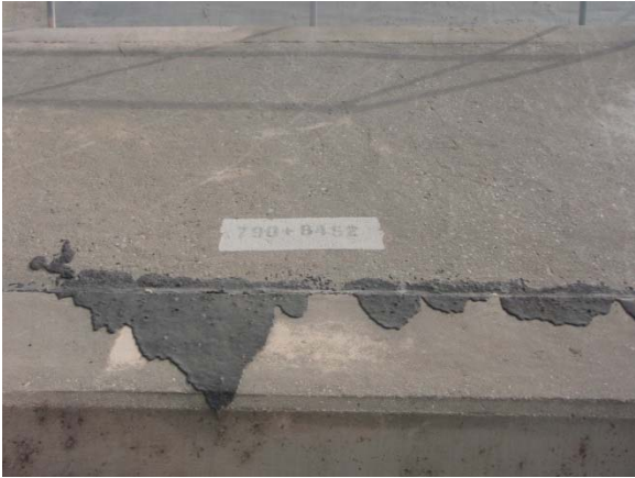
5. Markings near outfall
