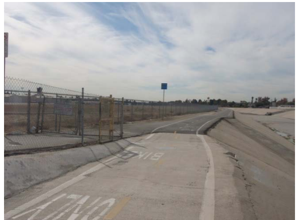
2. Looking South from top of outfall
