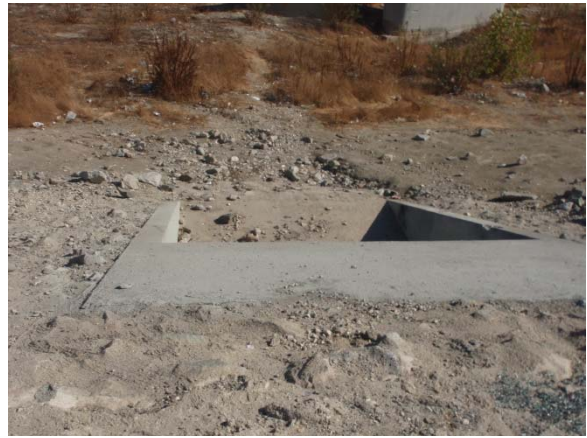
2. View from above outfall
