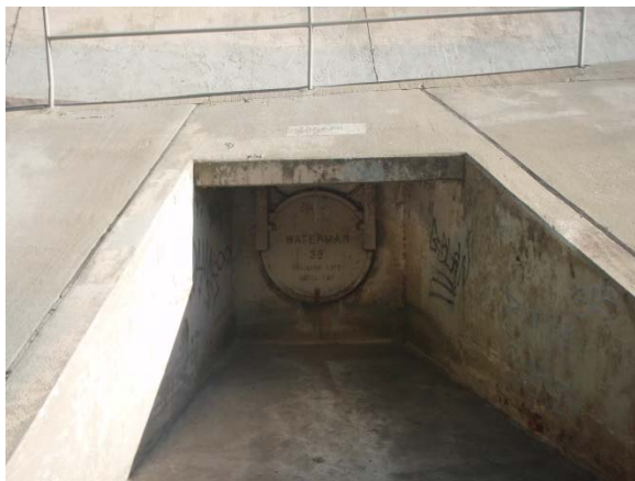
3. View of outfall
