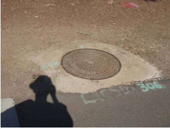
5. West manhole close up
