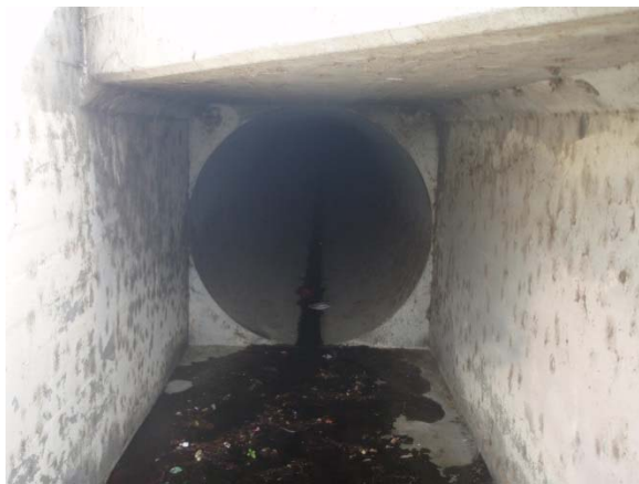
3. View of outfall
