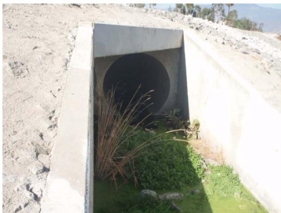
3. Close up view of outfall
