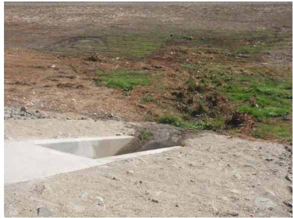
2. View looking down at outfall
