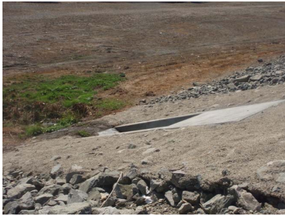
1. View looking down at outfall
