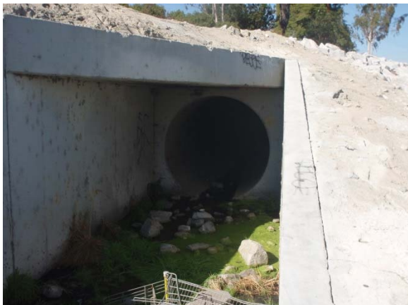
3. View of outfall
