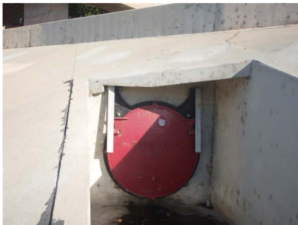
3. View of outfall
