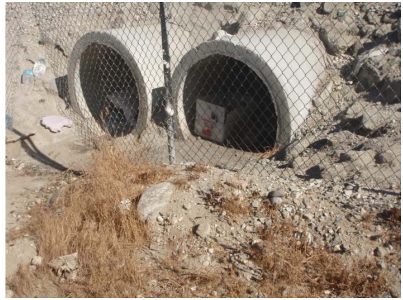
6. View showing possible habitation of pipes
