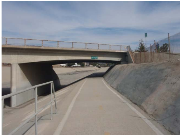
1. View of Lower Azusa bridge from top of outfall
