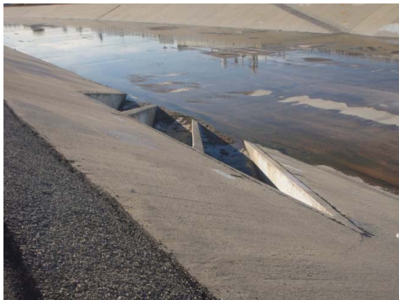
5. View of outfalls from bike path
