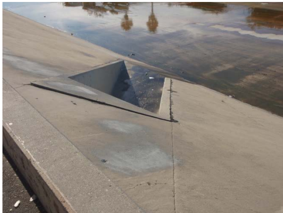
1. View of outfall from bike path
