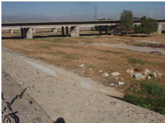
3. View of outfall looking towards Valley Blvd
