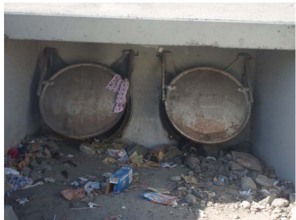
4. View of outfalls
