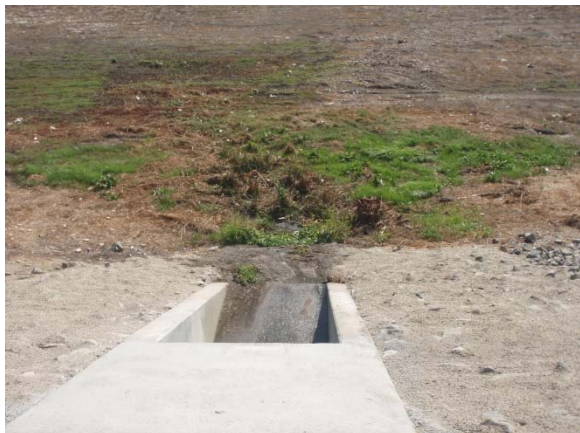
3. View looking down at outfall
