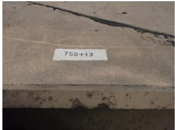
2. Marking on outfall
