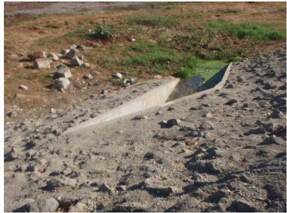
2. View from top of outfall
