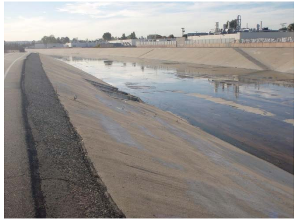
2. View looking South toward the three outfalls
