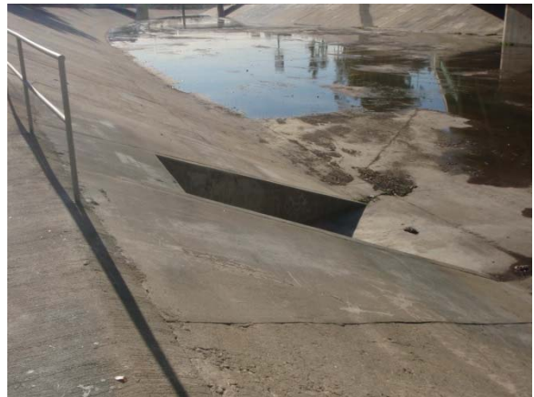
2. View of outfall
