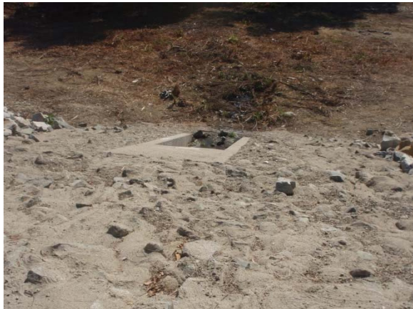
1. View looking down at outfall
