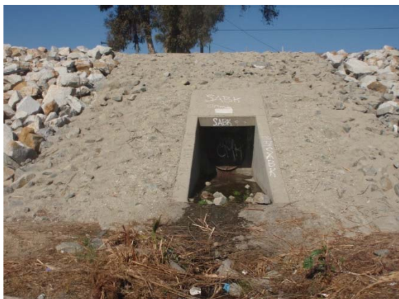
3. View of outfall
